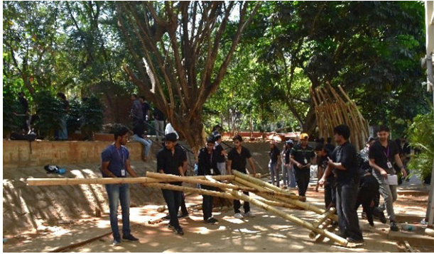
DAY 7- Assembling of main structure in the construction yard
